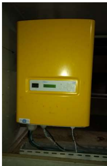
Figura 24 – Inversor CC/CA e CA/CC Sunny island Master
